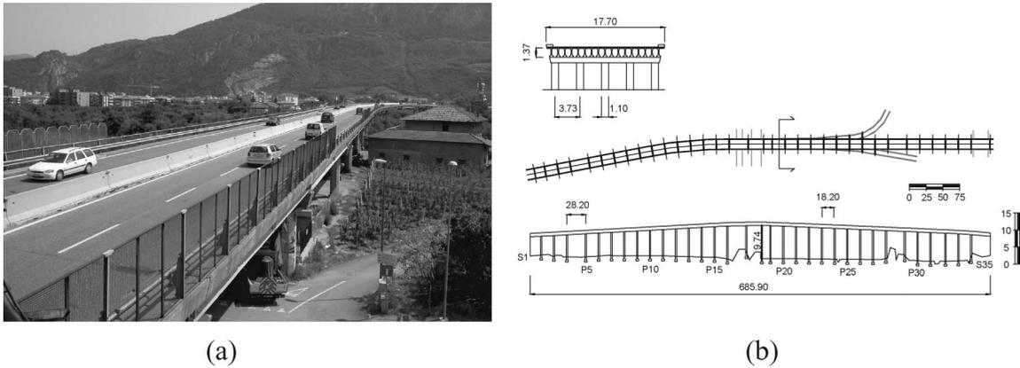
Figure 10. Canova Viaduct: (a) overview; (b) plan view, elevation and cross-section of the deck.
