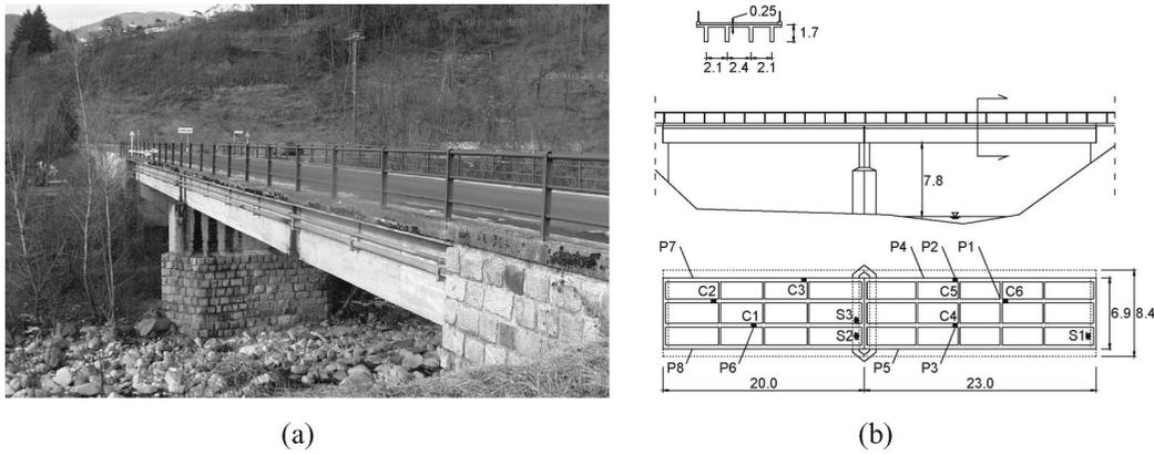
Figure 9. SP65 bridge on Maso river, near Carzano: (a) overview; (b) plan view, elevation and cross section of the deck.
