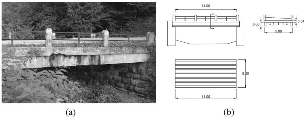
Figure 11. SP12 bridge on Vignola river: (a) overview; (b) plan view, elevation and cross-section of the deck.
